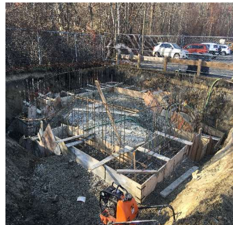
Steel Rebar in Place at Rail Trail
