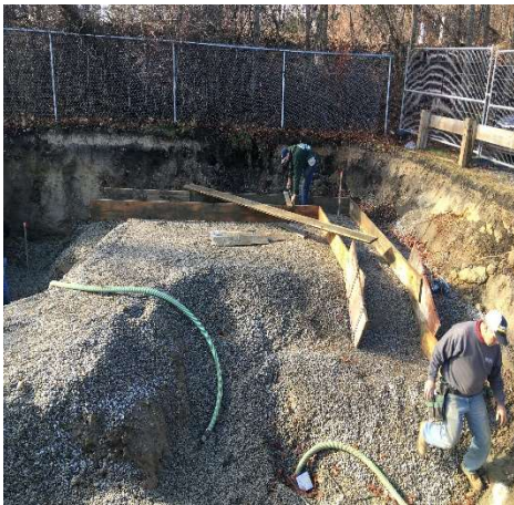
Placing Wooden Forms for Rebar Ties at Rail Trail
