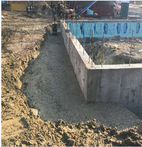
Rigid Insulation and De-Watering at Northland Road
