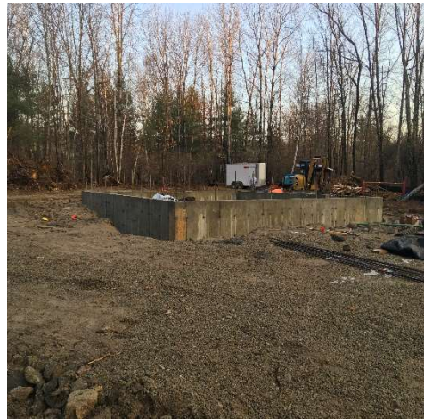
Foundation Walls in Place at Northland Road
