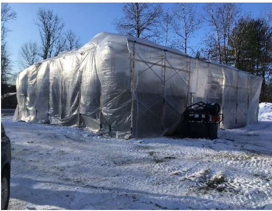
Building at Northland Road Tented for Masonry
