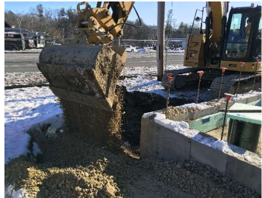
Structural Fill being Placed and Compacted
