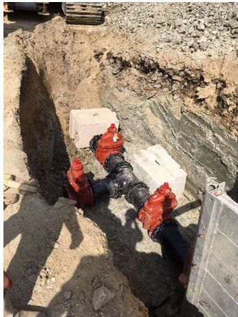
Gate valve installation for Lamson Road Crossing
