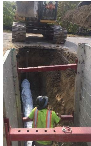
Water Main installation across Lamson Road
