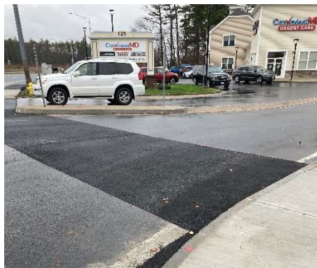
Pavement and sidewalk restoration at Convenient MD entrance
