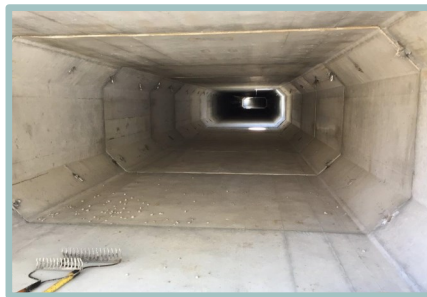
Inside the box culvert
