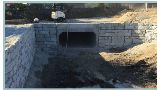
Box culvert outlet at Tuscan Village
