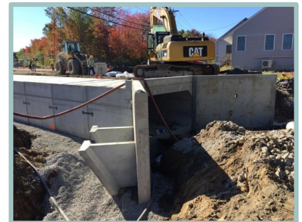
Box culvert inlet at Pleasant Street
