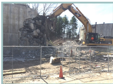
Demolition of the first sedimentation tank
