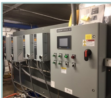
Domestic Variable Frequency Drives (VFD for pumps)
