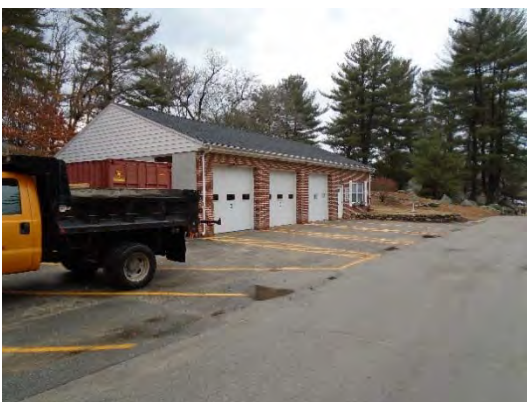
Existing administration/maintenance building.
