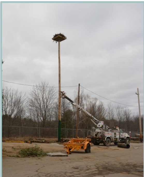
Pole set in concrete, 8 feet deep, predator guard (green) 8 feet high
