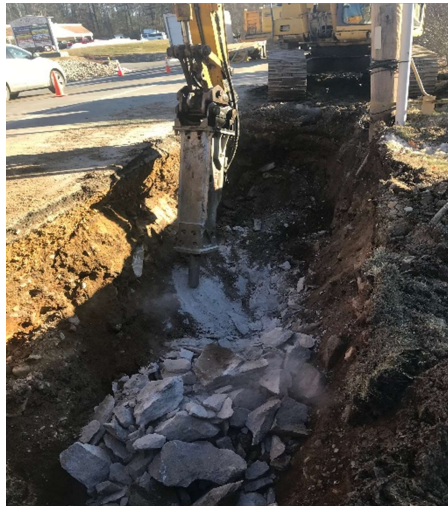
Ledge being Crushed for Pipe Installation
