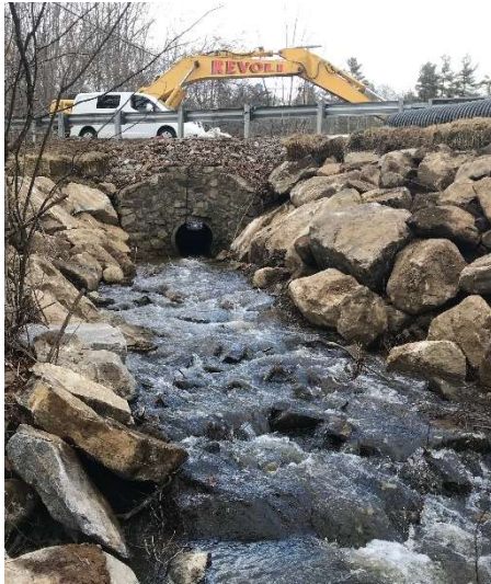
Outfall Wall Built at Culvert Crossing
