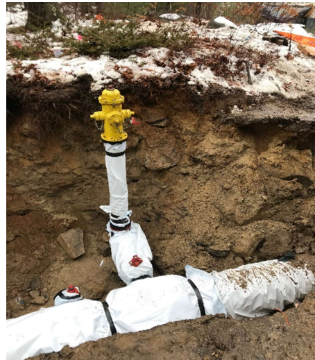
Fire Hydrant Installation
