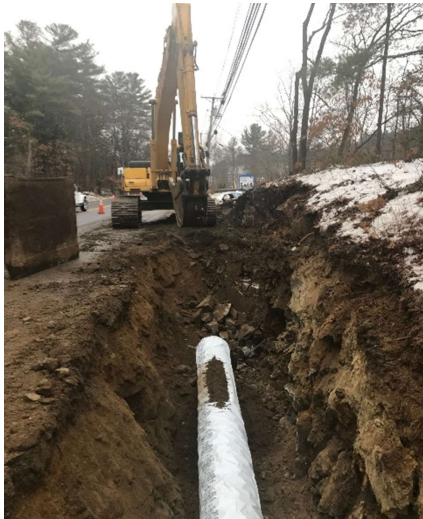
Backfilling Water Main Trench
