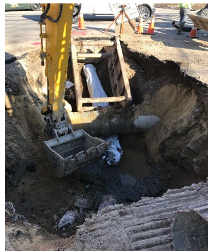
Water Main Install beneath Drain
