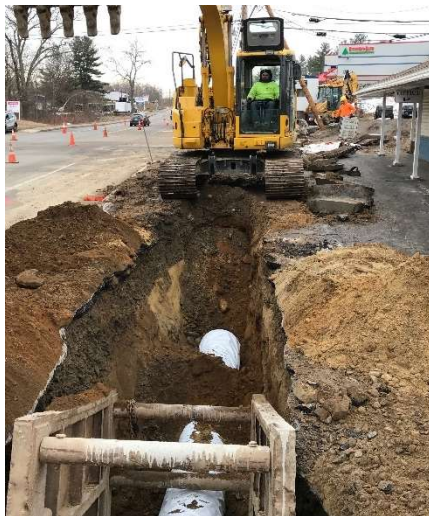
Water Main Installation
