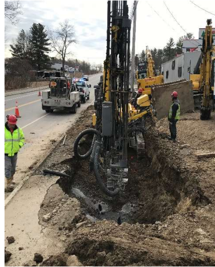
Drilling and Blasting Holes
