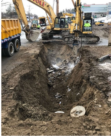
Hammering Rock within Water Main Trench
