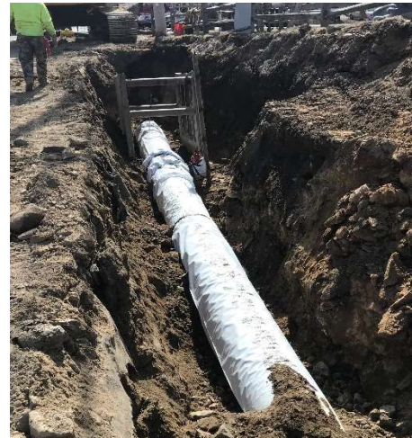
Water Main Installation
