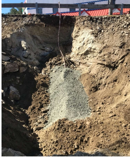
Water Service Stub to Cyr Lumber
