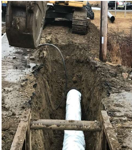
Water Main Installation
