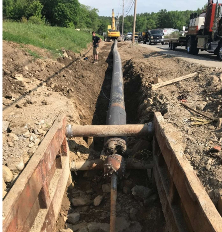
Directional Drill Head at Route 111
