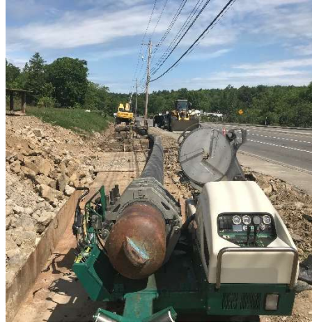
Thermal Fusion and Alignment of Pipe
