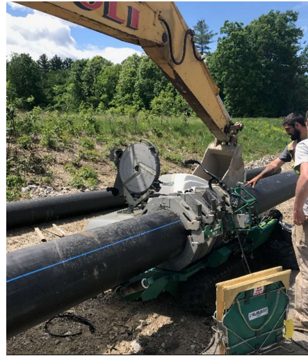
Thermal Fusion of HDPE Pipe
