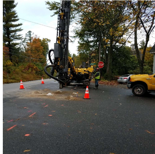
Preparation for Drilling and Blasting
