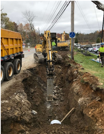
Preparation for Water Main Install
