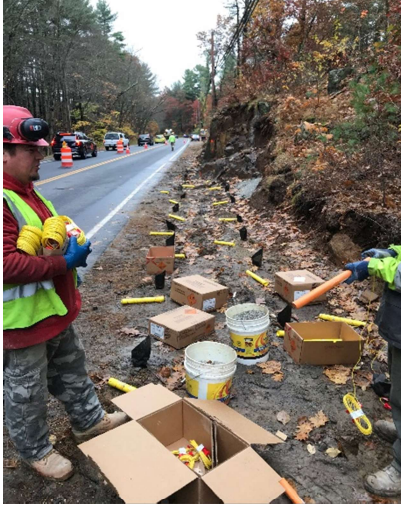
Blasting Preparation Along Route 28
