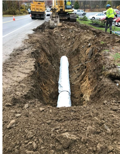
Water Main Installation Work Began
