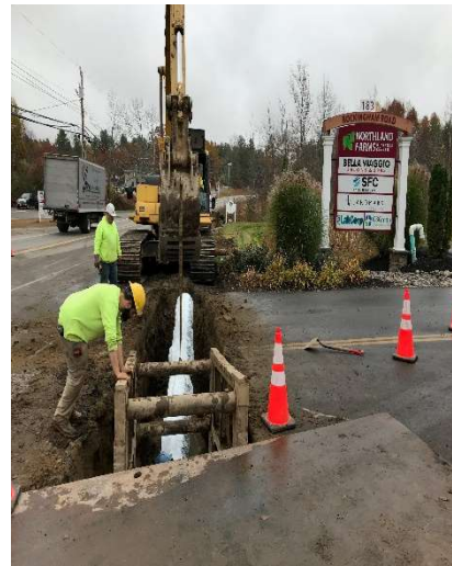
Water Main Installation at Driveway Crossing
