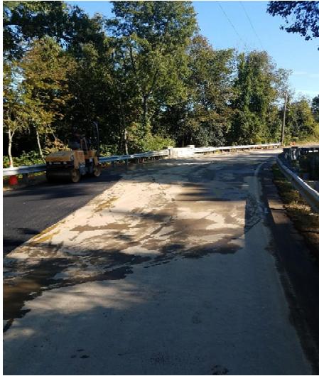
Trench Paving on Providence Hill Road
