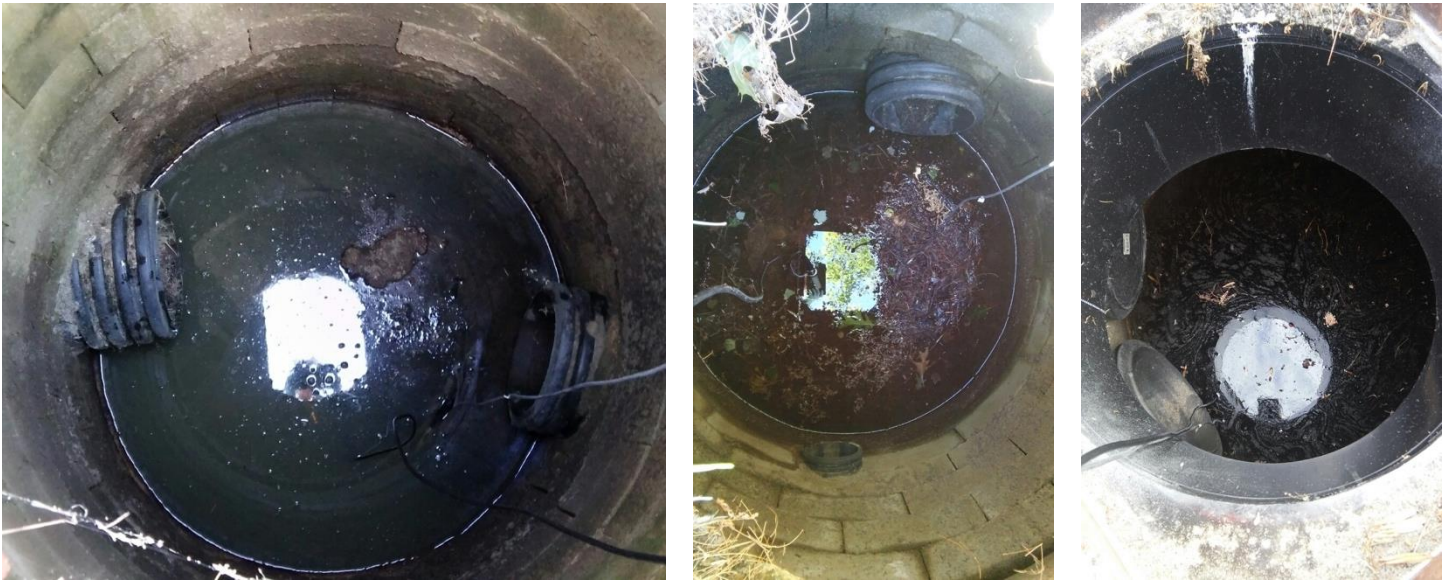
FIGURE 2. CB-3000 (left) during dry weather sampling showed evidence of dumping of some sort, perhaps dog feces, which would account for the E. coli concentration >2420 col/100 mL. CB-3001 (center) with minimal stormwater present, even after a 0.8" precipitation event the day prior. CB-3375 (right) during dry weather conditions.
