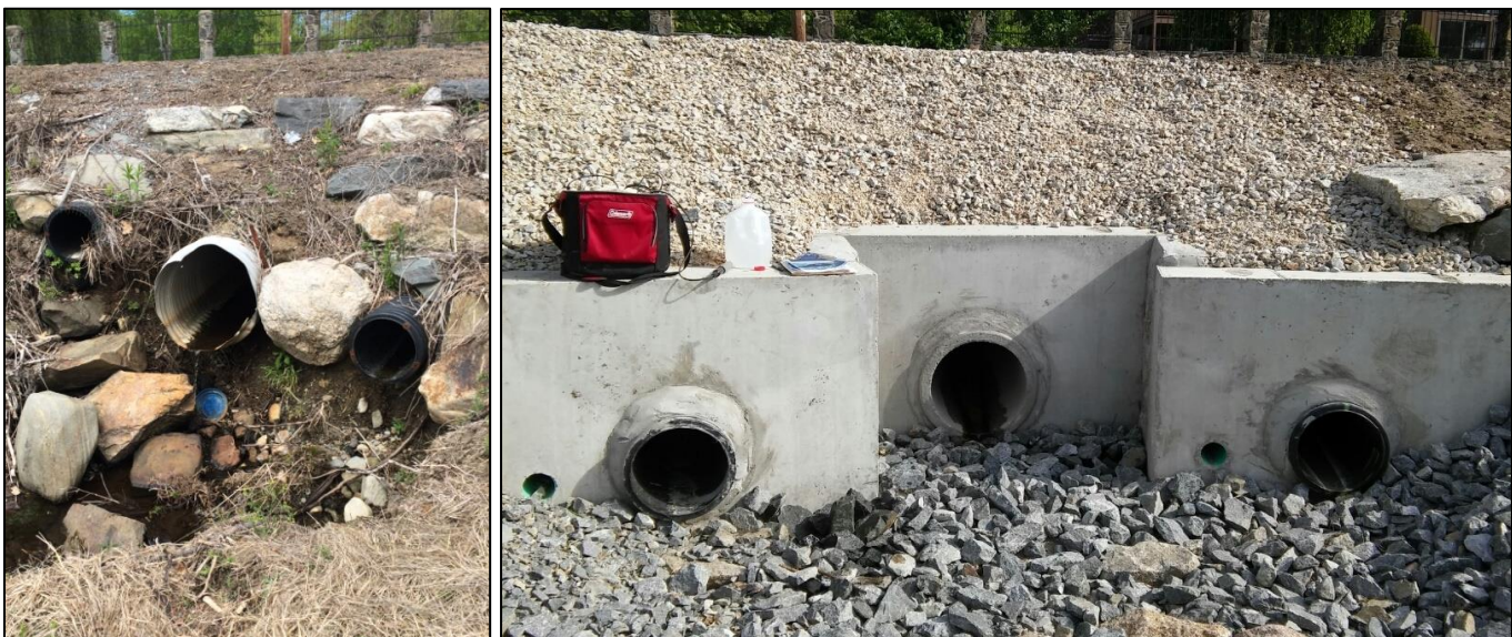
FIGURE 4. Before and after photos of culvert and headwall replacements at OF-0611 (left pipe) and 1906 (center pipe).
