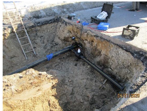
Gas main repair work
