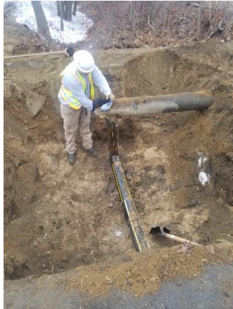
Gas main repair work
