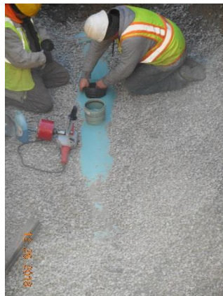
Sewer Service Installation
