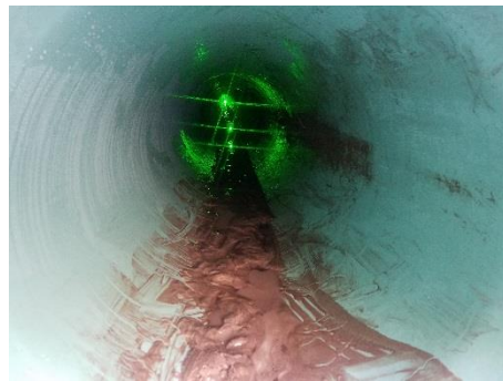
New Sewer Pipe Installation with Laser Level
