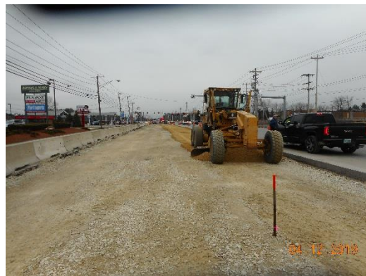
Fine Grading in Preparation for Paving
