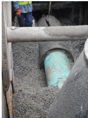
Sleeved Sewer Pipe Installation at Culvert Crossing
