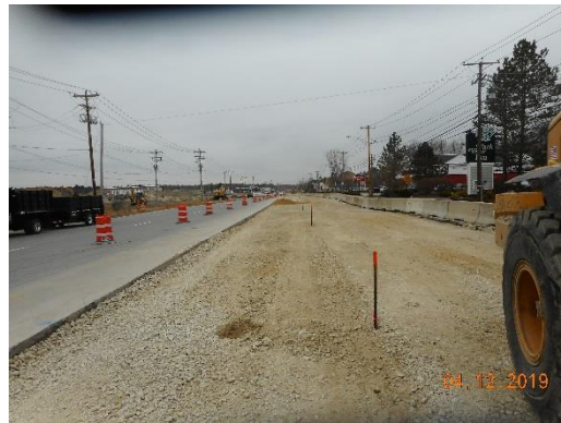
Fine Grading in Preparation for Paving
