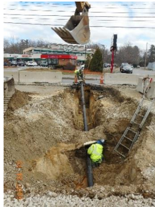
Fire Hydrant Branch Installation
