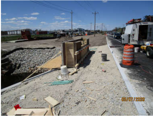
Concrete Guardrail Formwork (West)
