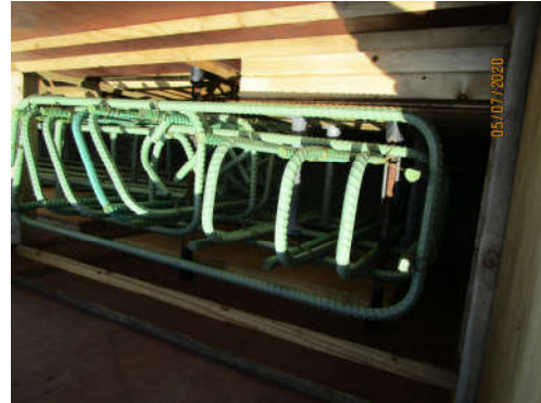
Guardrail Formwork Preparation
