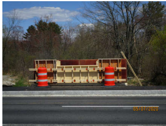
Concrete Guardrail Formwork (East)
