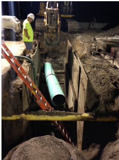
New Sewer Pipe Installation
