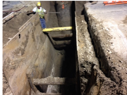
Trench Excavation for Sewer Manhole Coring
