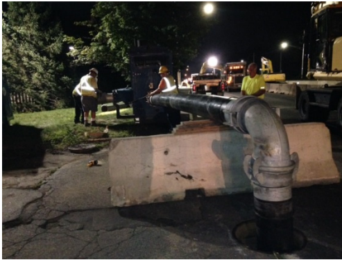
Existing Sewer Flow Bypassing
