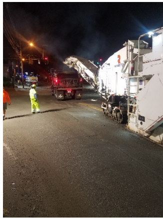
Pavement Milling
