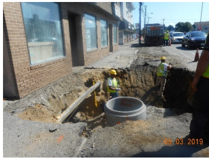
Catch Basin and Drain Installations
