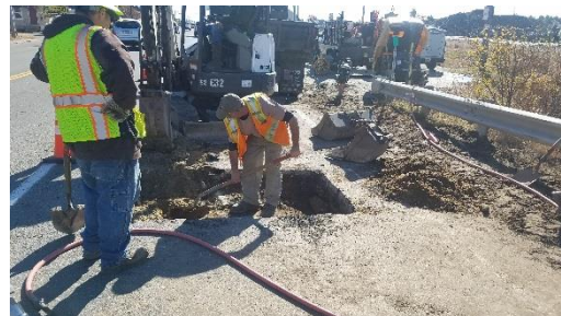
Test pit investigations at bridge location
