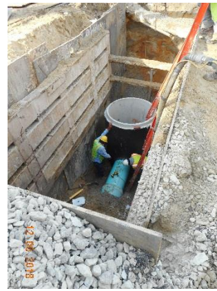
Sewer Manhole Installation
