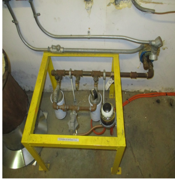
Oil supply piping. Note capped line.
