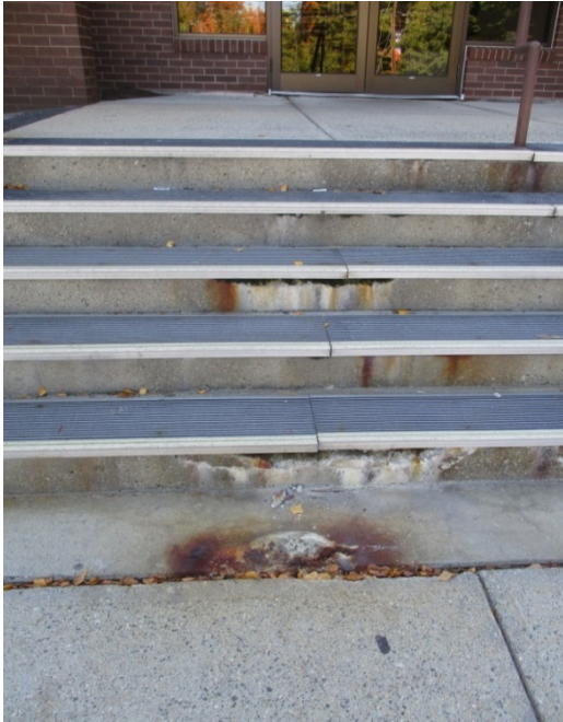
Concrete deterioration at main entrance stairs.
