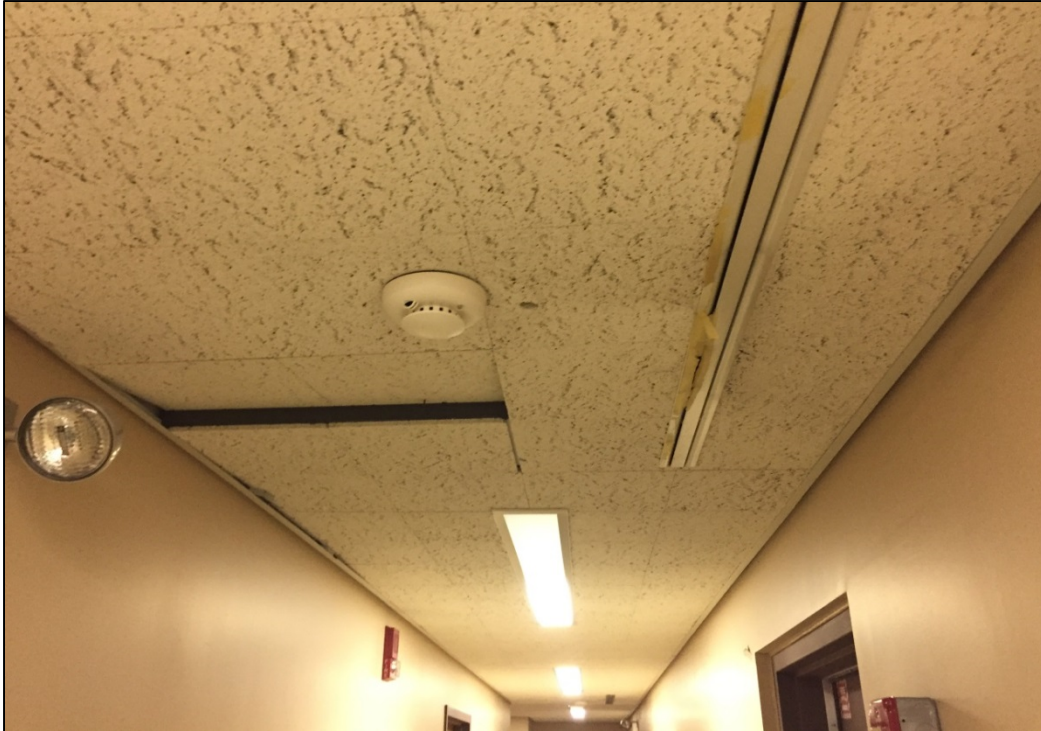
Spline-type acoustical ceiling. Unable to get tile back into place after maintenance.
