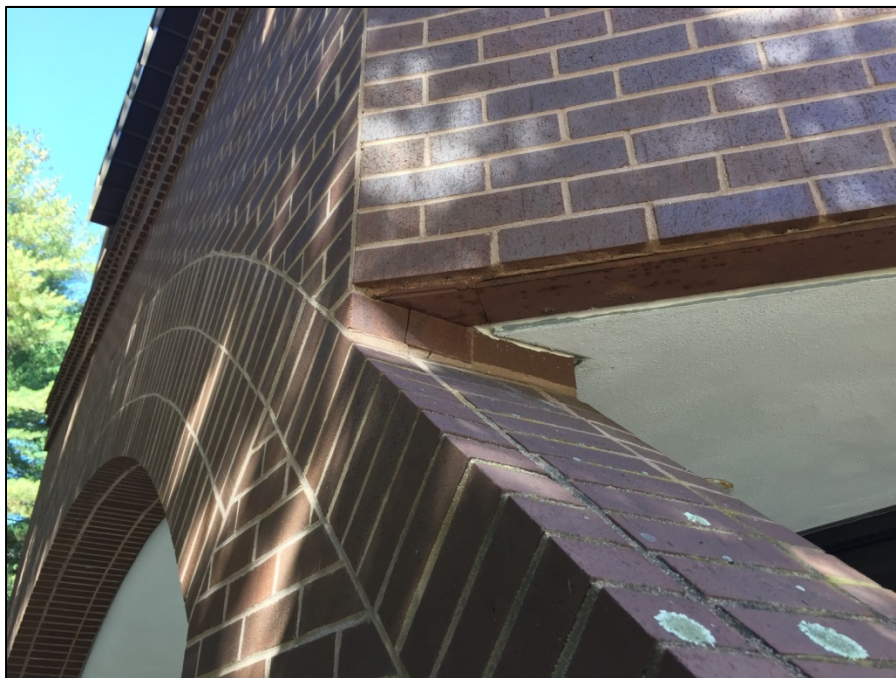
Steel lintel bearing on cracked brick.
