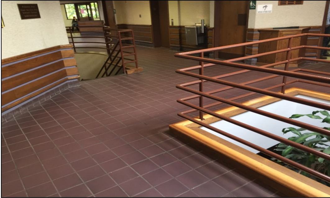
Guardrail around floor opening. Note excessive opening between horizontal rails.
