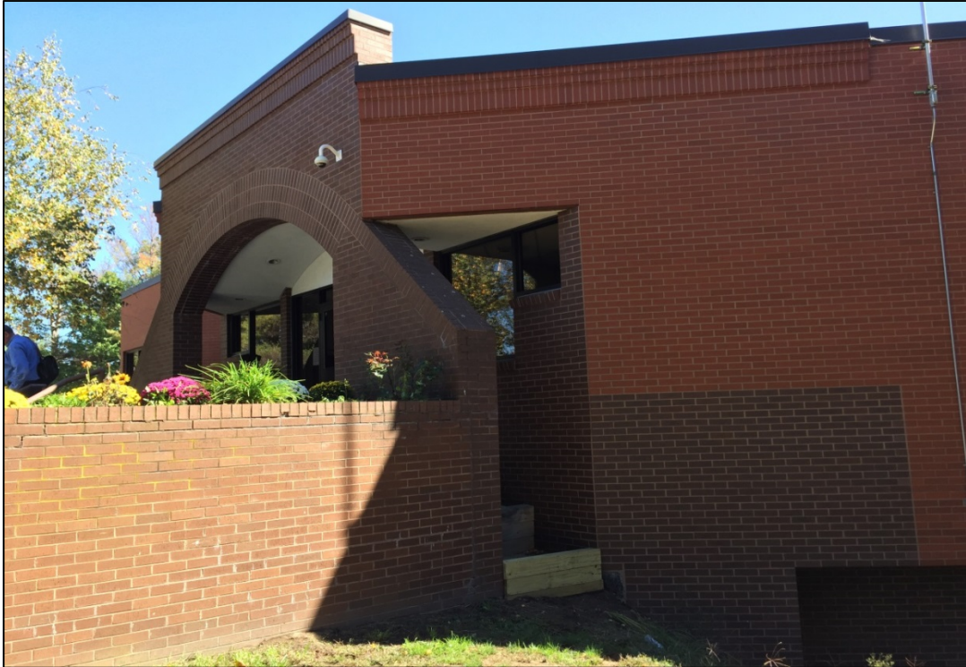
Missing mortar between bricks along planter. Wood timbers placed to retain soil and keep it from washing out adjacent to main entry.
