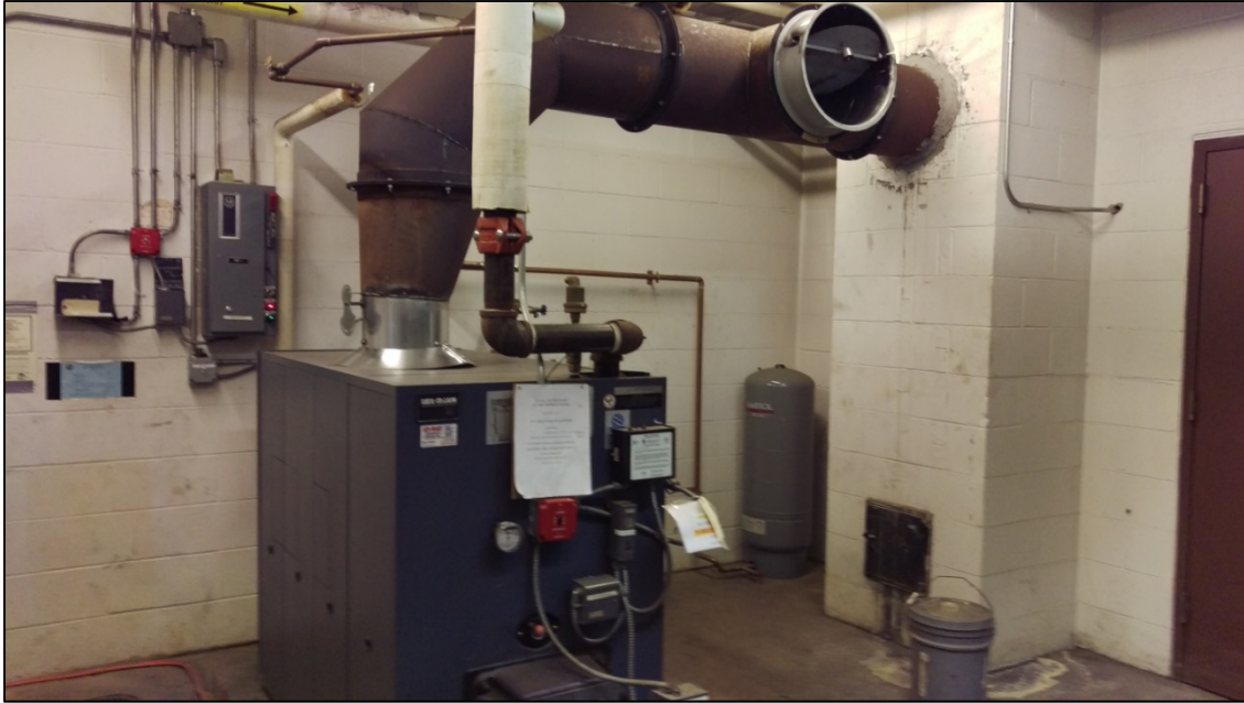
Oil-fired boiler.
