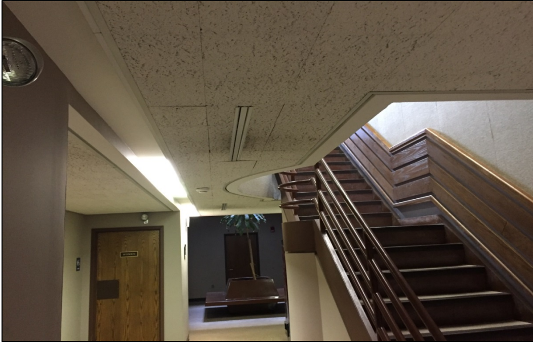
Staining on tiles around air vents.
