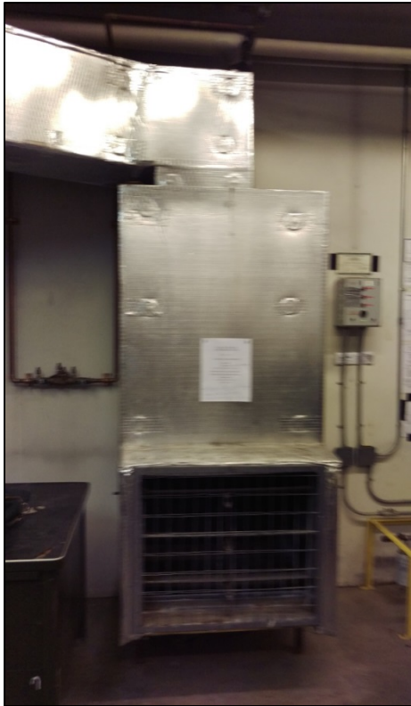
Combustion air duct.
