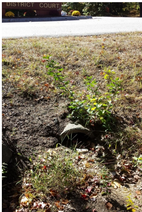
Culvert inlet at driveway entrance. Note sediment in swale.
