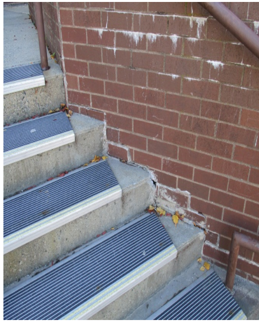
Concrete and brick deterioration at main entrance.
