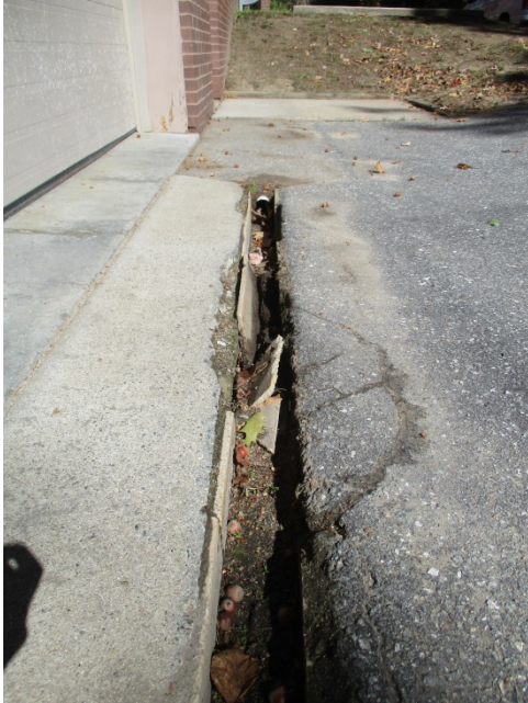
Trench drain on east side of Courthouse.
