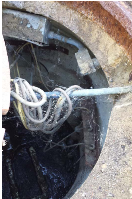
Pump station junction box and float rack.
