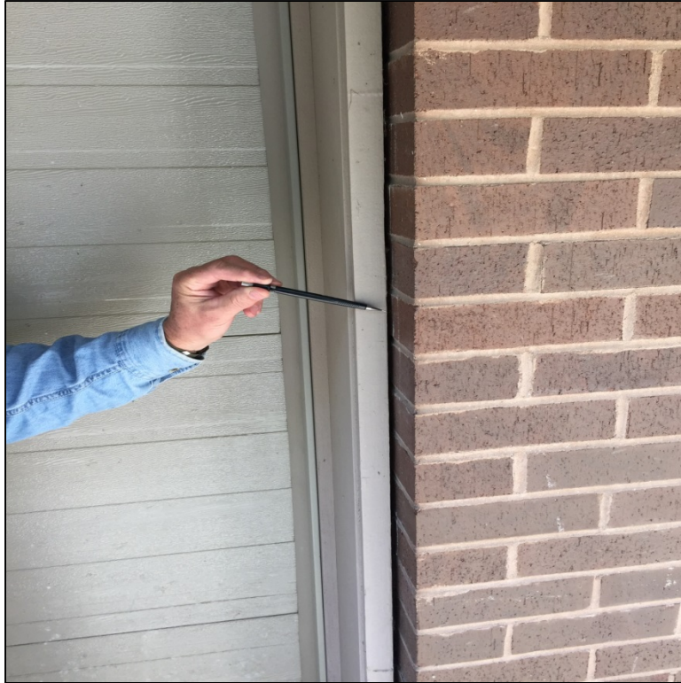
Missing caulking around door at judge's parking garage.
