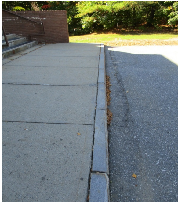
Displaced curbing.
