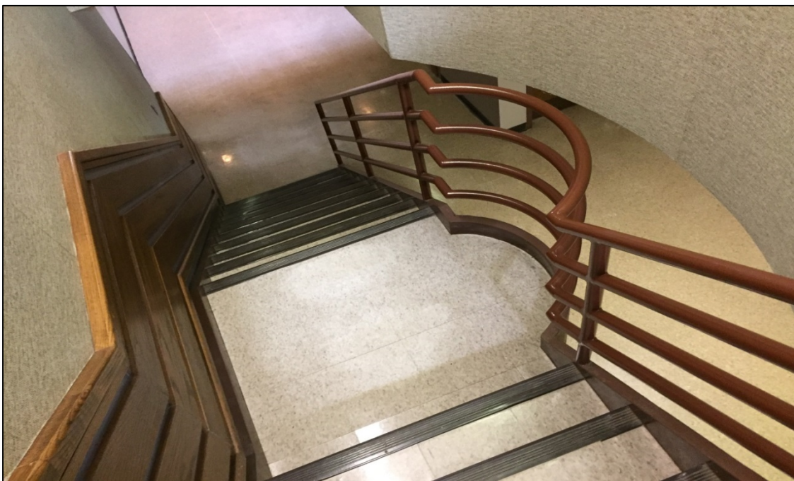
Main stairway from lobby. Note lack of proper handrail on either side and oversized openings in guardrail.
