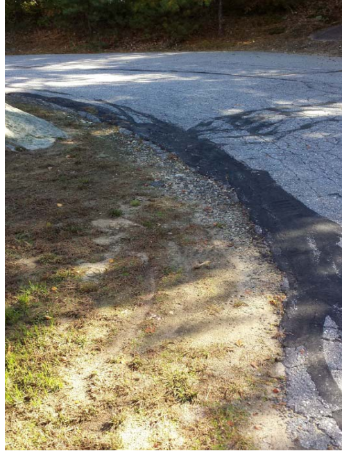
Failing pavement.
