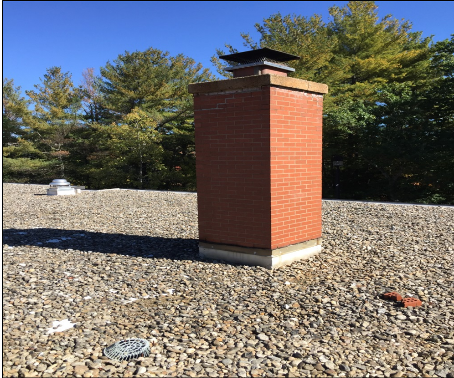
Top of chimney needs repointing and repairs to concrete cap.
