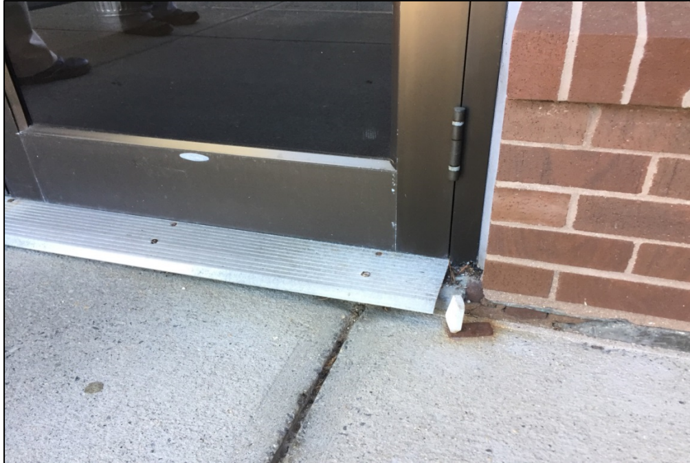
Slab has settled resulting in a raised sill at main entry.
