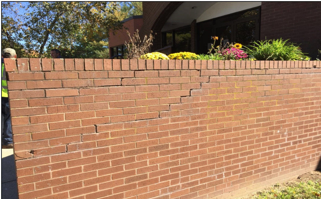
Planters at main entry require re-pointing repairs.
