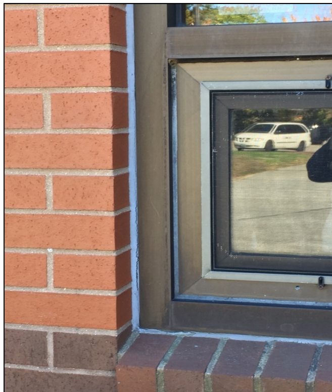
Caulking around window units is starting to fail.
