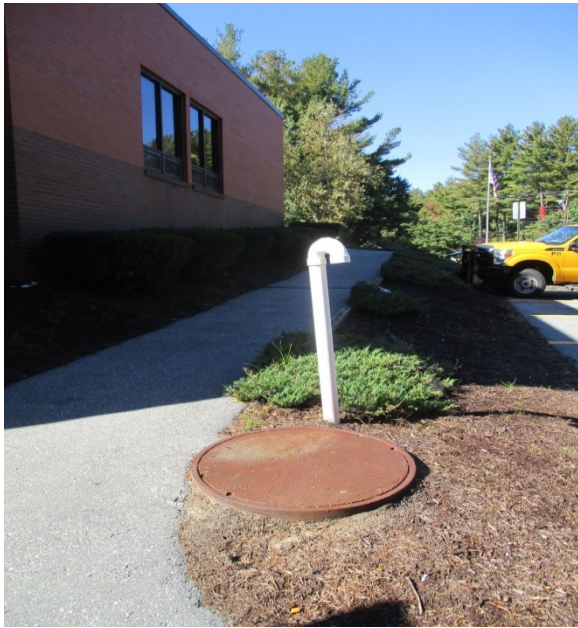
Pump station and vent pipe.
