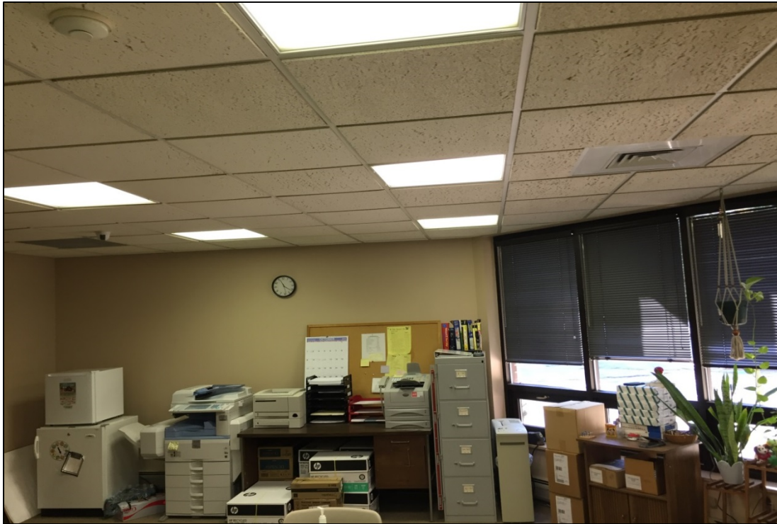
Grid-type acoustical ceiling in probation department.
