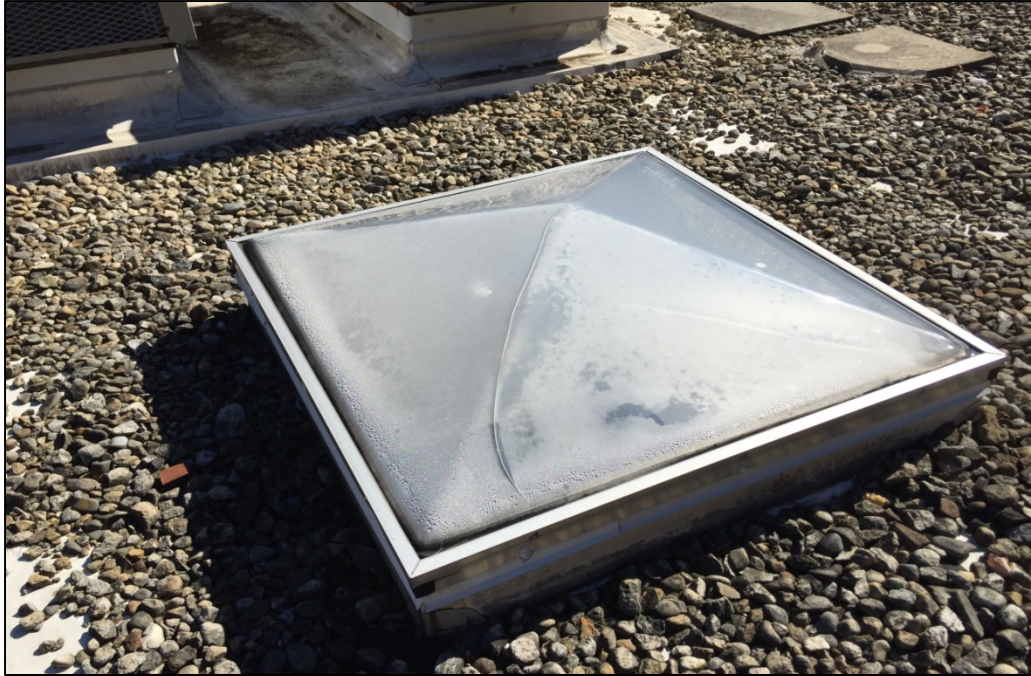
Note build-up of condensation in skylight.
