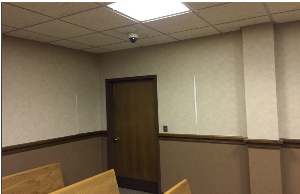
Peeling wallpaper and grid-type acoustical ceiling in juvenile hearing room.
