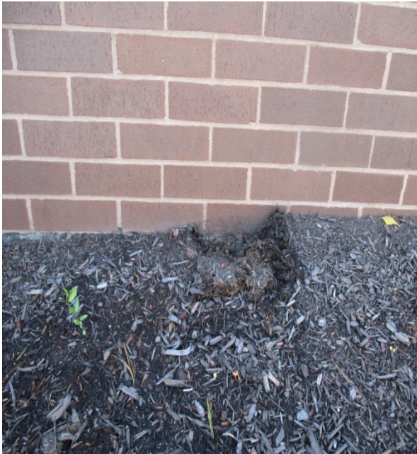
Mulch piled over masonry weeps.
