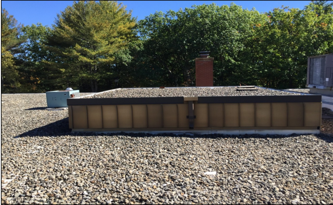
Raised roof section over courtroom ceiling coffers. Note single drain scupper in foreground.
