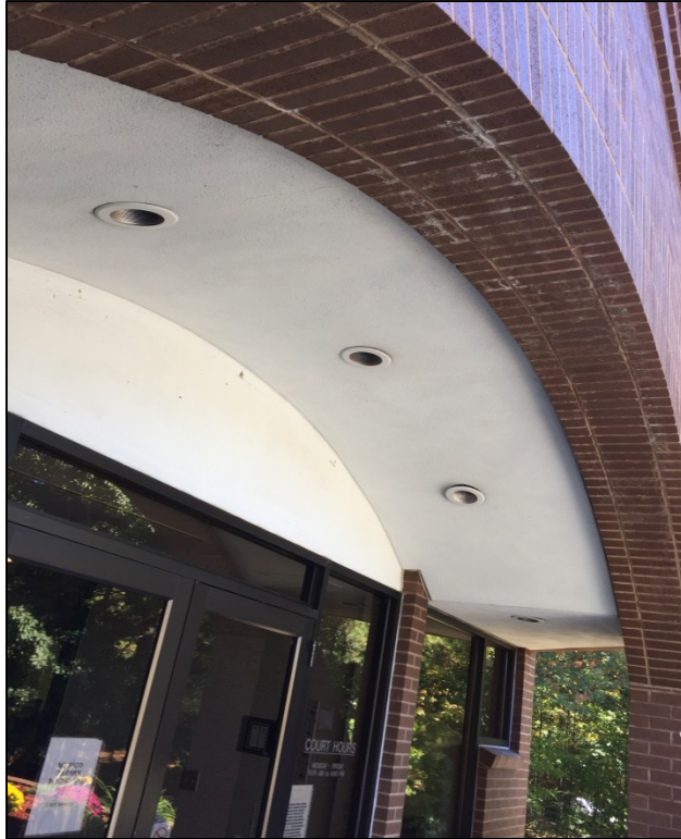
Efflorescence on brickwork under archway at main entry.
