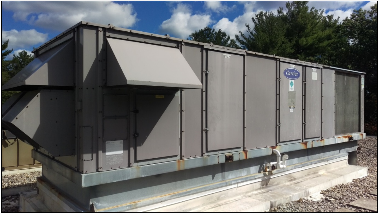
Large roof mounted air handling unit. Main unit for Level 1.
