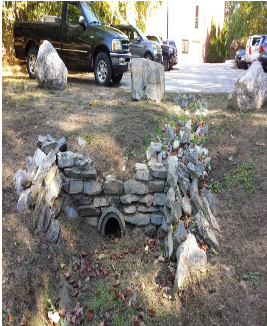
Obstructed drainage pipe outlet and crumbling retaining wall.
