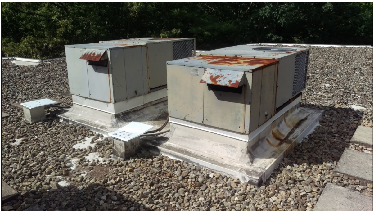
Roof mounted air handling units serving the lower level.
