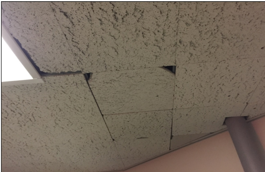
Broken corners/edges and misaligned tiles on spline-type acoustical ceiling.
