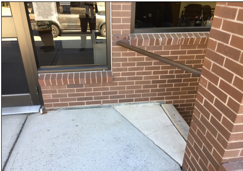
Slab at main entry is settling as material is washed out from under slab. Note settlement crack.
