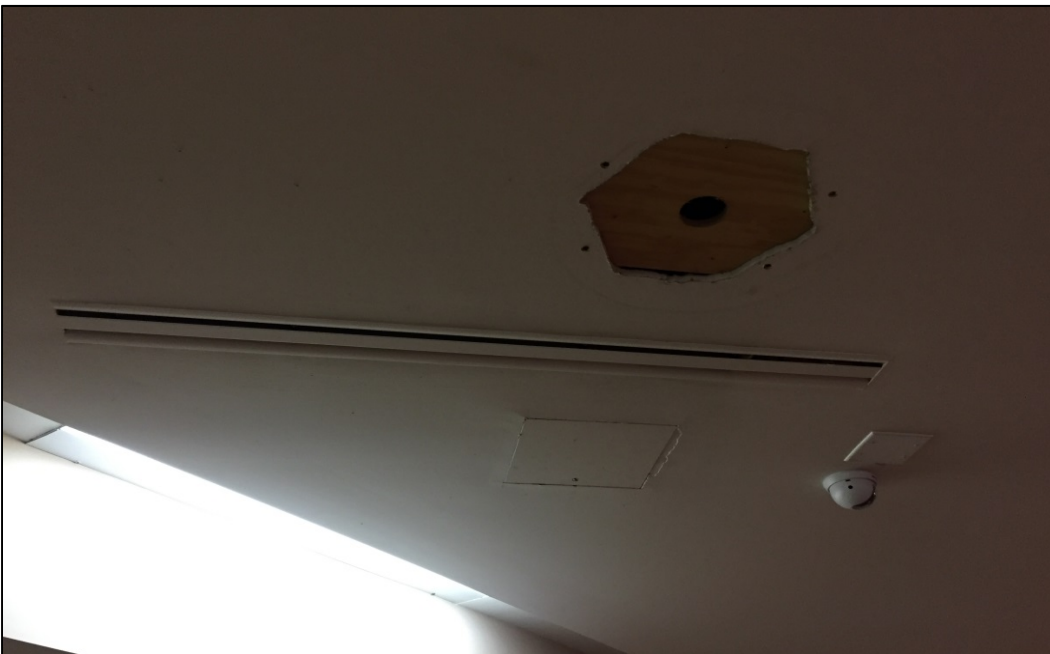
Ceiling in courtroom requires patching.
