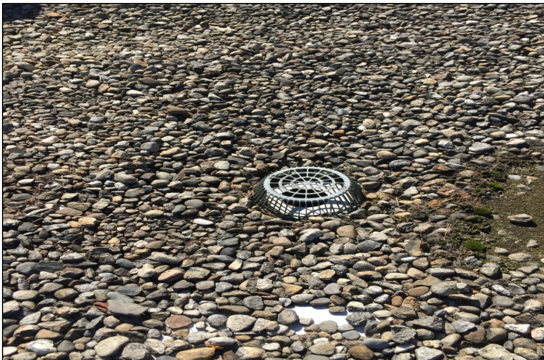
Typical roof drain with a build-up of debris around strainer.
