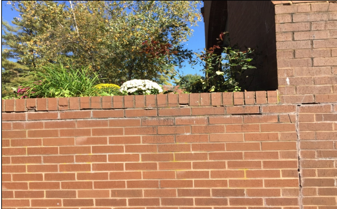
Poor condition of planters at main entry. Note caulking in expansion joint is failing.
