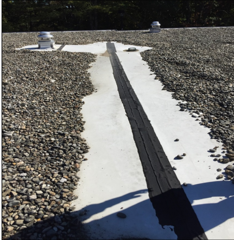
Stone ballasted EPDM or TPO roof membrane. Seams have been re-stripped.
