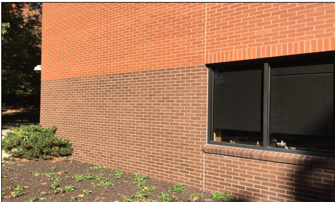
Typical brick façade; caulking in expansion joint in good condition; mulch blocking weeps.
