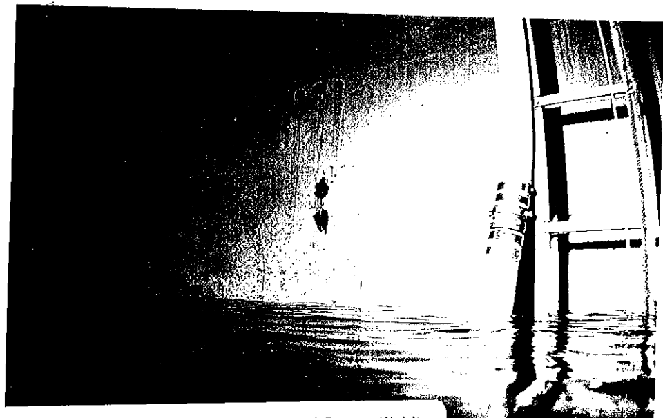
59. Failed Coating and Corrosion Found Within Lowest Thirteen Panels
