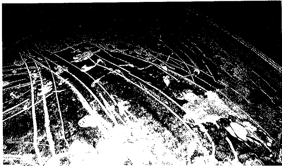
27. Stained Floor Coating Found With Good Adhesion Value After Cleaning
