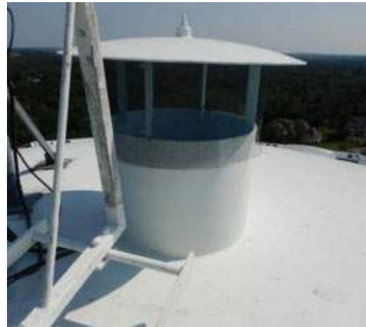
Figure 5-2 Finial vent atop the Lawrence Road Tank (photo by USCI)
