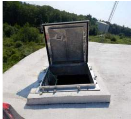
Figure 5-3 Roof hatch atop the Spicket Hill Tank (photo by USCI)
