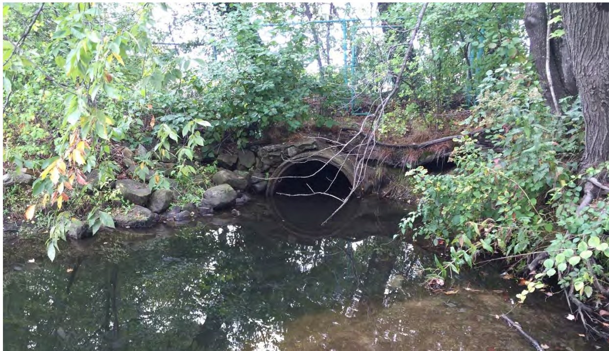
Location 7A: Area shows the lack of flow around a culverted area.
