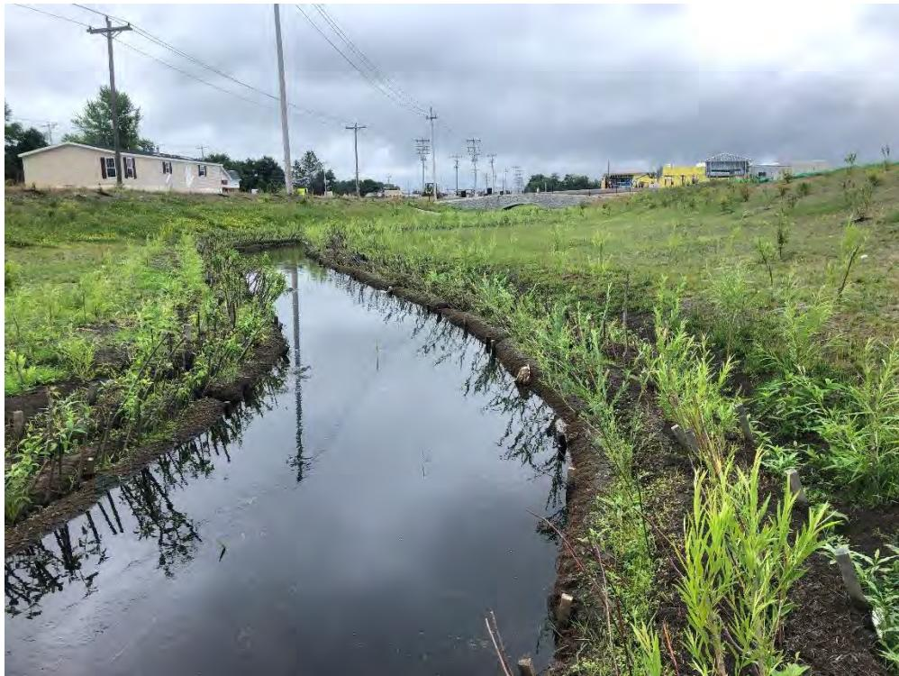
**Photo 15&16: June 2020, dormant cuttings installed in May are sprouting**
