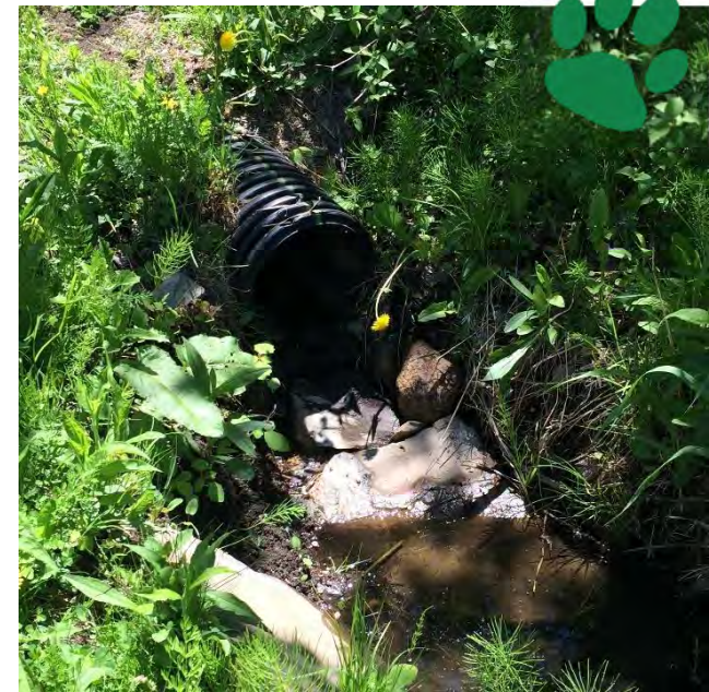
Water from storm drains empties directly to waterbodies through outfall pipes, such as the one pictured above.
