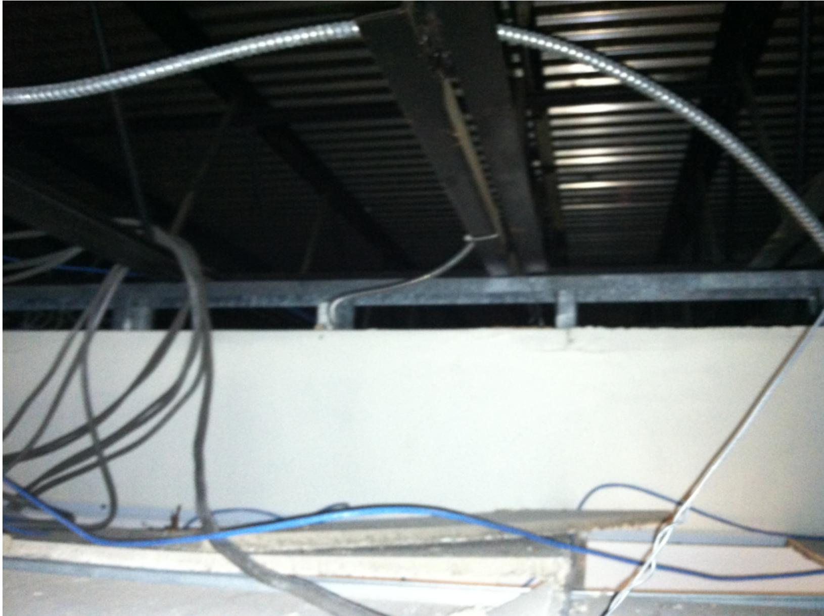
EXISTING STUD WALL TO BE EXTENDED AND SEALED AGAINST EXISTING DECK
