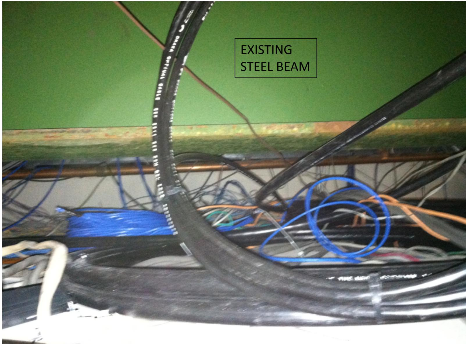
EXISTING COPPER HEATING PIPE TO BE RELOCATED IS SEEN BELOW THE EXISTING STEEL BEAM. ALL WIRING TO BE ORGANIZED USING J-HOOKS
