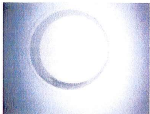
The coating on the interior face of the shell manhole is in excellent condition with only silt staining noted on the manhole neck
