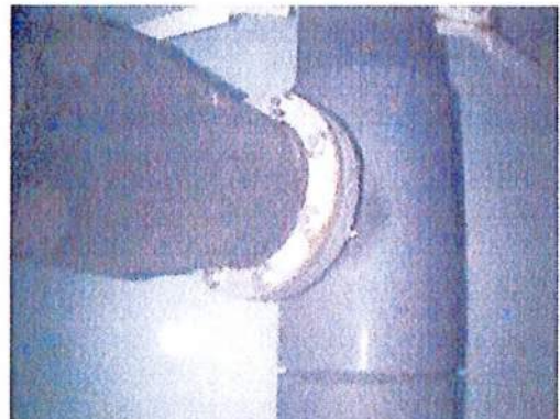
Shows typical corrosion on the mixing system flanges
