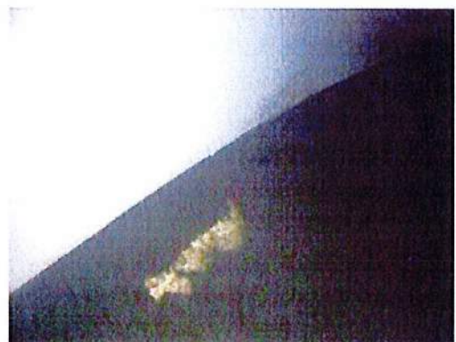
No coating degradation was observed where the silt layer was moved to expose the floor
