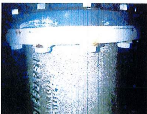
Scattered light to medium grade rust is present throughout the mixing system connections
