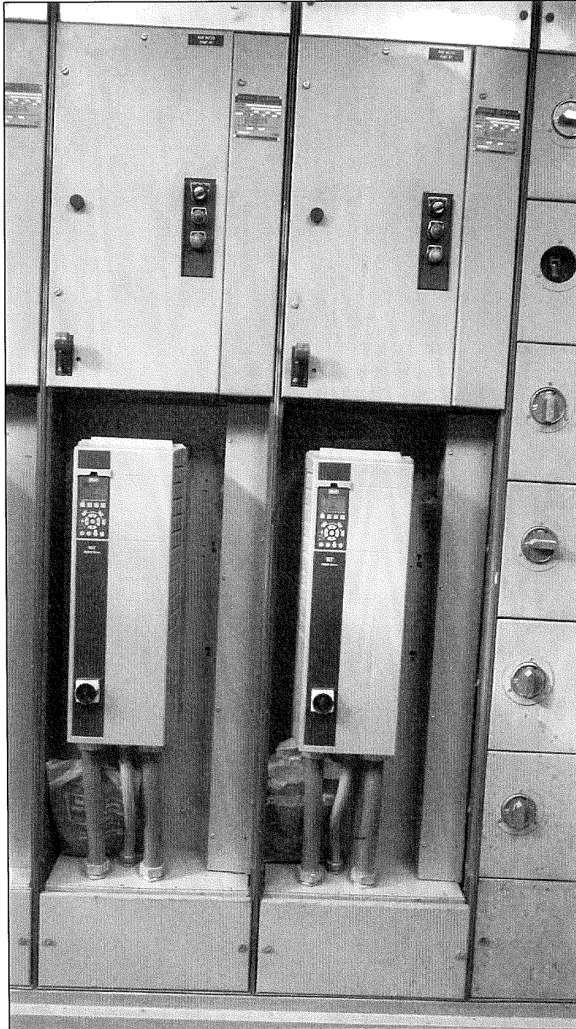
FIGURE 1 CANOBIE LAKE RAW WATER PUMP VFD (EXAMPLE)
