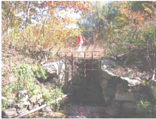
Culvert north of Willow Street
