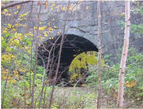
Historic stone arch bridge
