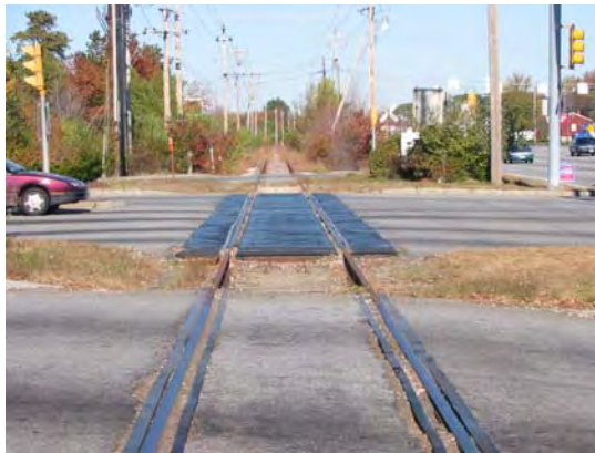
Rail crossing at Rockingham Boulevard
