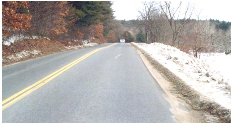
Ash Street looking east
