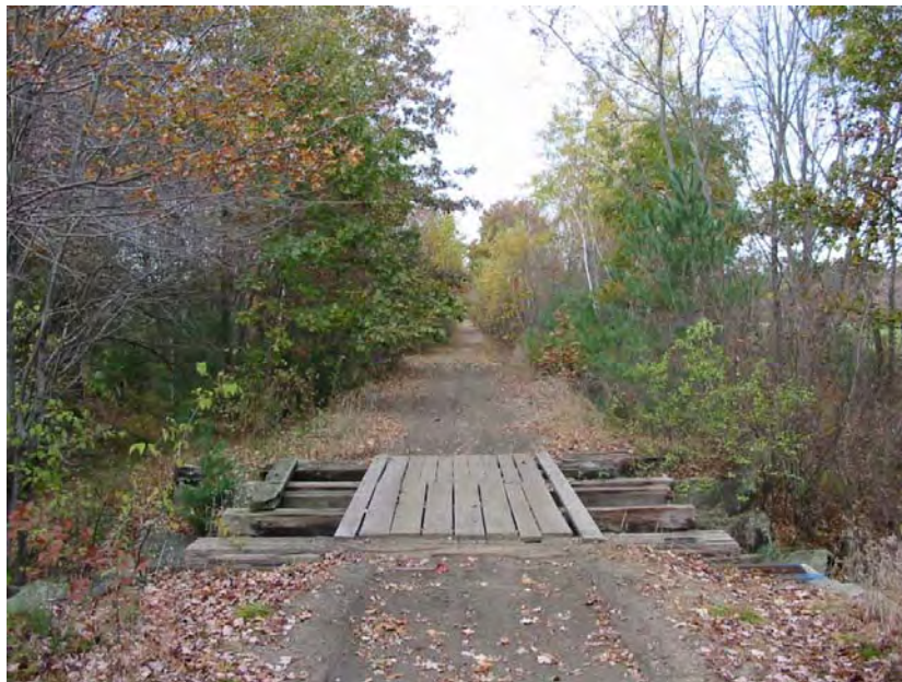
Rail bridge over Shields Brook in Londonderry.
