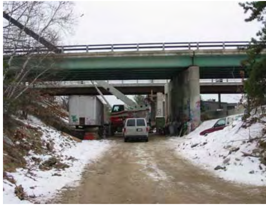
The abandoned rail corridor passes under I-293
