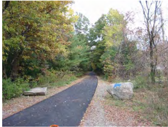
Existing paved path in Derry
