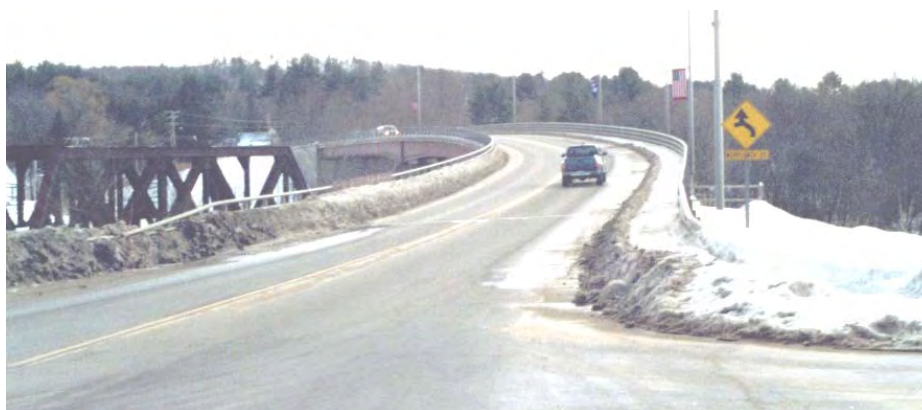
Main Street Bridge in Hooksett
