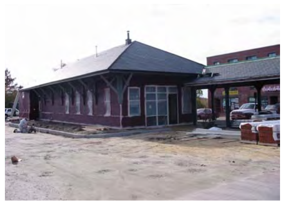
Derry Depot under renovation in October 2002
