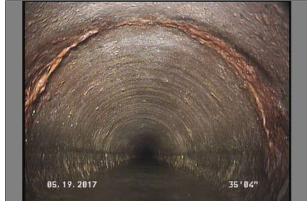
Photo: 112_4A, MPEG #: 050517_1, 00:01:24 35.35FT, Infiltration Weeper, from 08 to 04 o'clock, within 8 inches of joint: YES
