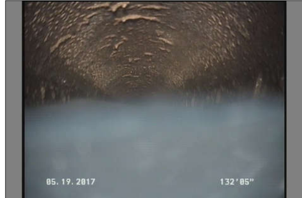
Photo: 115_6A, MPEG #: 050517_1, 00:04:03 132.25FT, Water Level, Sag in pipe, 50 %of cross sectional area
