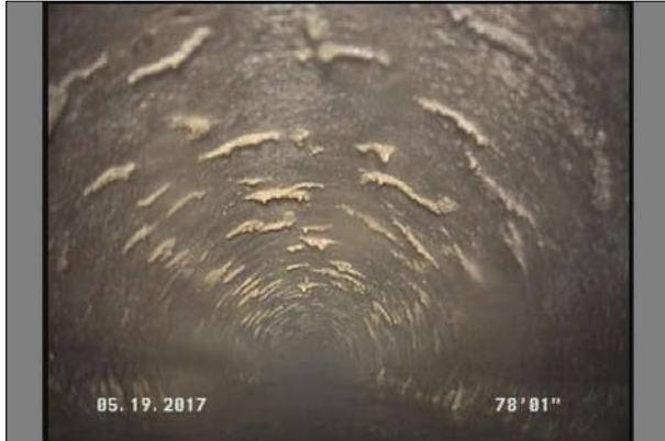
Photo: 115_5A, MPEG #: 050517_1, 00:02:52 75.35FT, Deposits Attached Grease, 10 %of cross sectional area, from 08 to 04 o'clock, , within 8 inches of joint: YES, Start
