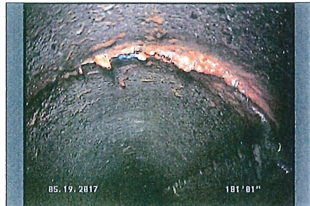
Photo: 1503 - 1504__19052017031300_A.JPG 181.1FT, Deposits Attached Encrustation, 5 %of cross sectional area, from 01 to 04 o'clock, , within 8 inches of joint: YES
