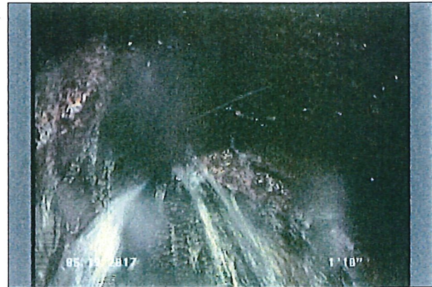
Photo: 1505 - 1506__19052017041639_A.JPG 2.85FT, Broken, from 08 to 04 o'clock, within 8 inches of joint: YES
