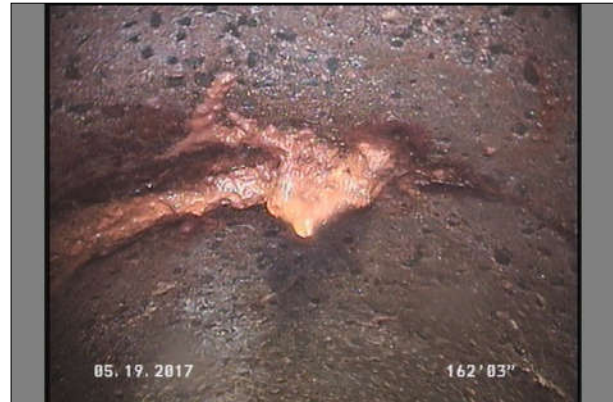
Photo: 116_12A, MPEG #: 050517_1, 00:07:06 162.25FT, Surface Reinforcement Visible, from 08 to 01 o'clock, within 8 inches of joint: NO
