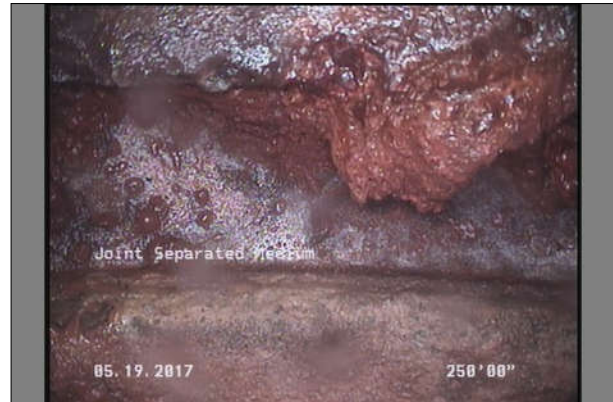
Photo: 116_18A, MPEG #: 050517_1, 00:10:33 250FT, Joint Separated Medium
