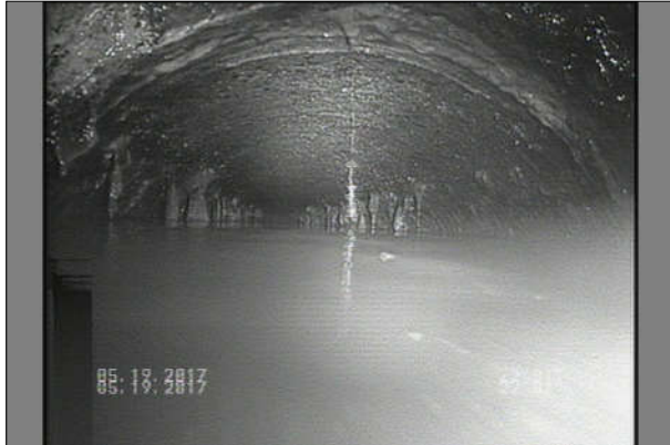
Photo: 114_5A, MPEG #: 050517_1, 00:02:11 22.1FT, Infiltration Dripper, from 11 to 01 o'clock, within 8 inches of joint: YES
