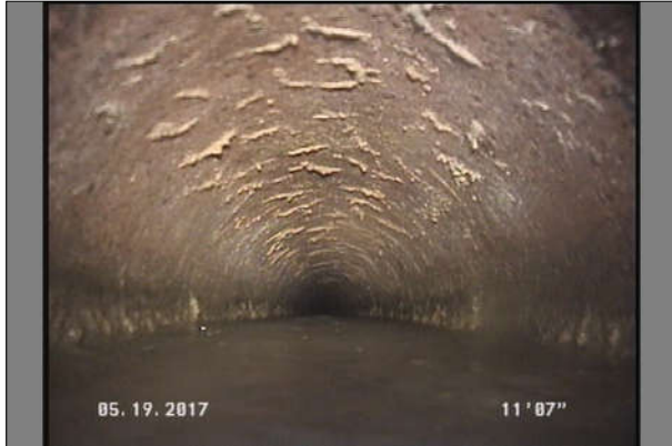
Photo: 116_3A, MPEG #: 050517_1, 00:00:50 8.8FT, Deposits Attached Grease, 5 %of cross sectional area, from 08 to 04 o'clock, , within 8 inches of joint: YES, Start
