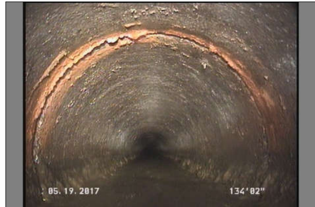
Photo: 116_10A, MPEG #: 050517_1, 00:06:01 134.2FT, Infiltration Weeper, from 08 to 04 o'clock, within 8 inches of joint: YES
