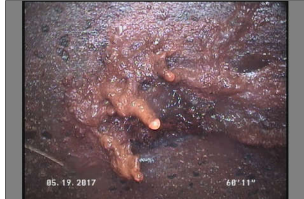
Photo: 116_4A, MPEG #: 050517_1, 00:02:36 60.9FT, Infiltration Dripper, from 01 to 02 o'clock, within 8 inches of joint: NO
