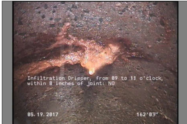
Photo: 116_11A, MPEG #: 050517_1, 00:06:47 162.25FT, Infiltration Dripper, from 09 to 11 o'clock, within 8 inches of joint: NO
