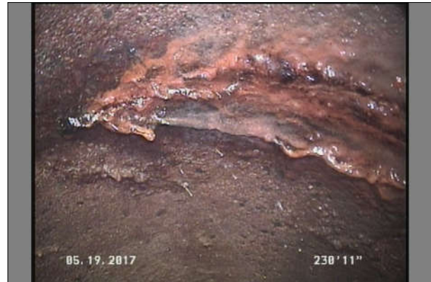
Photo: 112_6A, MPEG #: 050517_1, 00:05:55 233.65FT, Crack Circumferential, from 12 to 04 o'clock, within 8 inches of joint: NO
