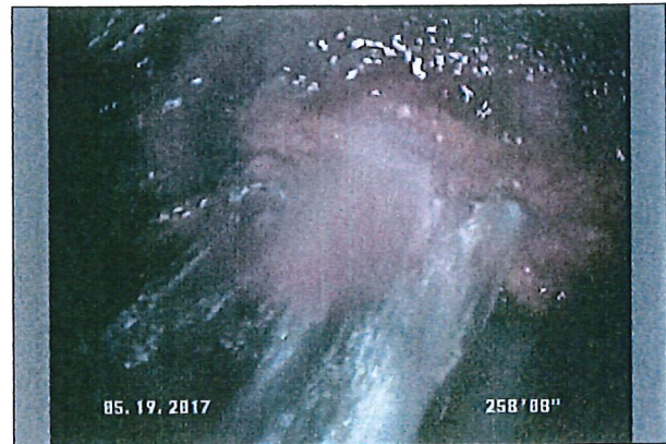
Photo: 1503 - 1504__19052017032239_A.JPG 258.7FT, Fracture Circumferential, from 08 to 04 o'clock, within 8 inches of joint: YES
