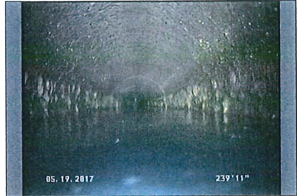
Photo: 1503 - 1504__19052017031940_A.JPG 239.2FT, Deposits Attached Grease, 10 %of cross sectional area, from 08 to 04 o'clock, , within 8 inches of joint: YES, Start
