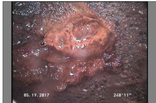
Photo: 116_14A, MPEG #: 050517_1, 00:09:12 240.95FT, Infiltration Dripper, from 10 to 11 o'clock, within 8 inches of joint: NO
