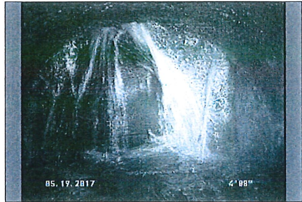
Photo: 1505 - 1506__19052017041724_A.JPG 2.05FT, Infiltration Gusher, from 08 to 04 o'clock, within 8 inches of joint: YES
