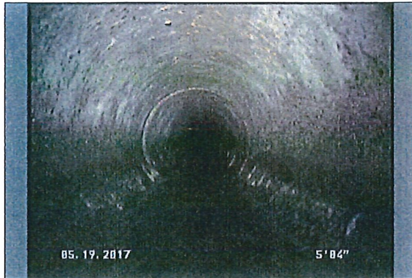
Photo: 1503 - 1504__19052017030805_A.JPG 5.05FT, Deposits Attached Grease, 10 %of cross sectional area, from 08 to 04 o'clock, , within 8 inches of joint: YES, Start
