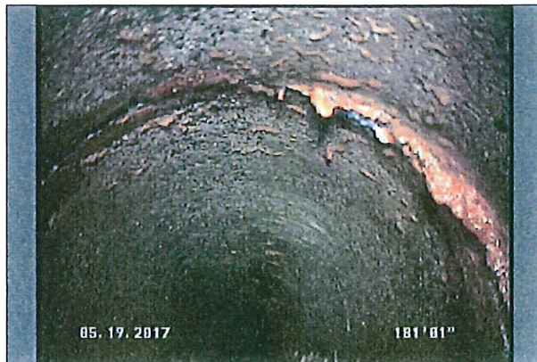
Photo: 1503 - 1504__19052017031224_A.JPG 181.1FT, Infiltration Dripper, from 08 to 04 o'clock, within 8 inches of joint: YES
