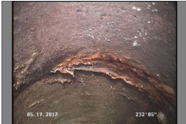
Photo: 112_5A, MPEG #: 050517_1, 00:05:19 232.4FT, Infiltration Dripper, from 12 to 04 o'clock, within 8 inches of joint: NO
