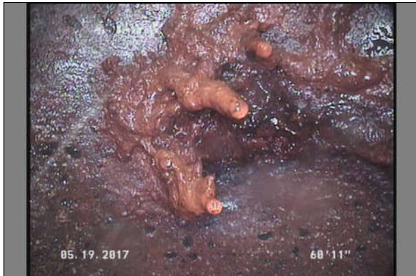
Photo: 116_5A, MPEG #: 050517_1, 00:03:10 60.9FT, Surface Reinforcement Corroded, from 01 to 02 o'clock, within 8 inches of joint: NO
