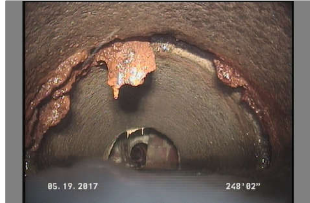
Photo: 116_16A, MPEG #: 050517_1, 00:09:47 248.2FT, Infiltration Dripper, from 08 to 04 o'clock, within 8 inches of joint: YES
