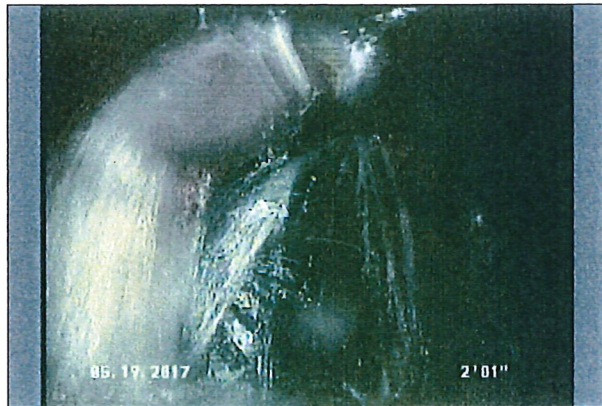
Photo: 1505 - 1506__19052017041556_A.JPG 2.05FT, Deformed, 30 %
