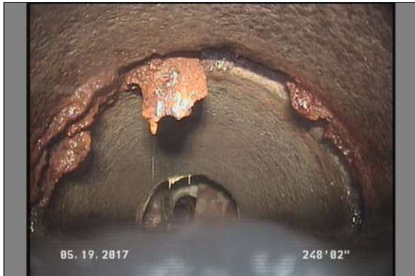
Photo: 116_17A, MPEG #: 050517_1, 00:09:58 248.2FT, Deposits Attached Encrustation, 10 %of cross sectional area, from 08 to 04 o'clock, , within 8 inches of joint: YES
