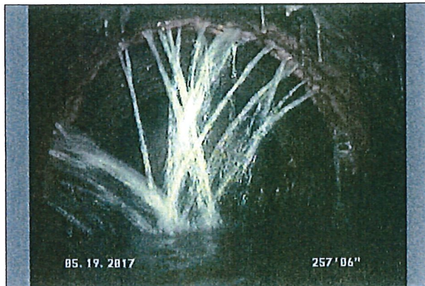
Photo: 1503 - 1504__19052017032051_A.JPG 258.7FT, Infiltration Gusher, from 08 to 04 o'clock, within 8 inches of joint: YES
