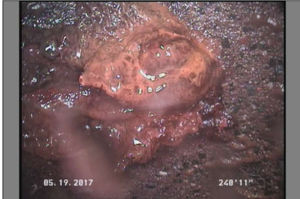
Photo: 116_15A, MPEG #: 050517_1, 00:09:21 240.95FT, Deposits Attached Encrustation, 5 %of cross sectional area, from 09 to 11 o'clock, , within 8 inches of joint: NO
