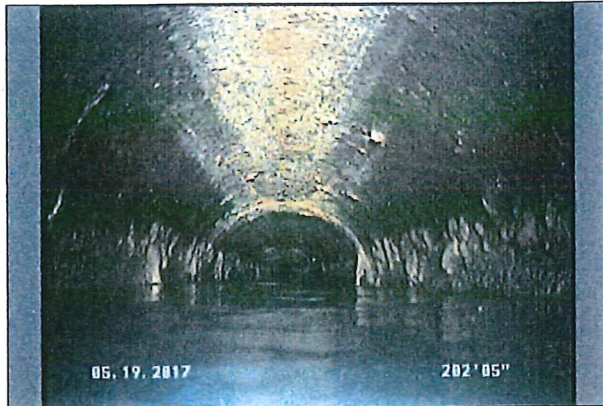
Photo: 1503 - 1504__19052017031355_A.JPG 202.45FT, Water Level, Sag in pipe, 60 %of cross sectional area
