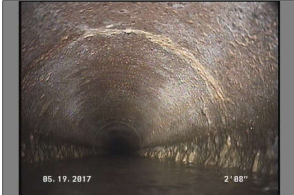
Photo: 112_3A, MPEG #: 050517_1, 00:00:34 0FT, Deposits Attached Grease, 10 %of cross sectional area, from 08 to 04 o'clock, , within 8 inches of joint: YES, Start
