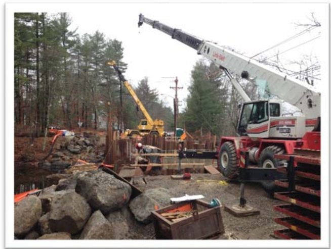
Removing Remaining Forms from the East Abutment Looking West
