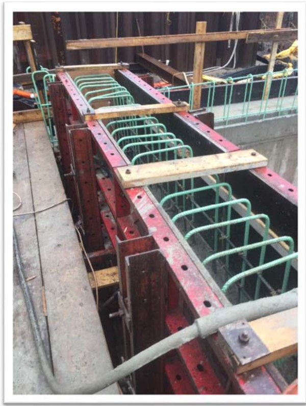
Pouring Concrete for the New East Abutment Wingwalls Looking West
