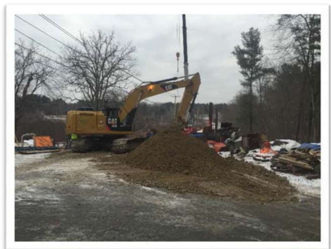
Backfill Material Behind West Abutment Looking East
