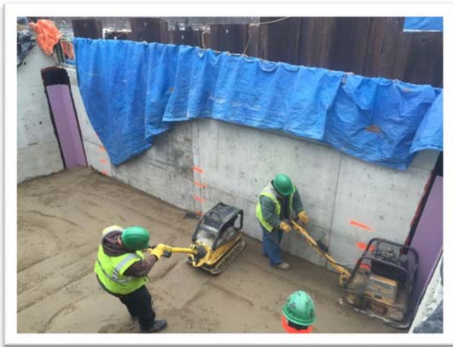
Compacting Backfill Material Behind West Abutment Looking East
