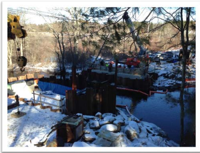
Work Area - Looking East
