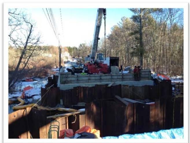
Forming the East Abutment Backwall - Looking East
