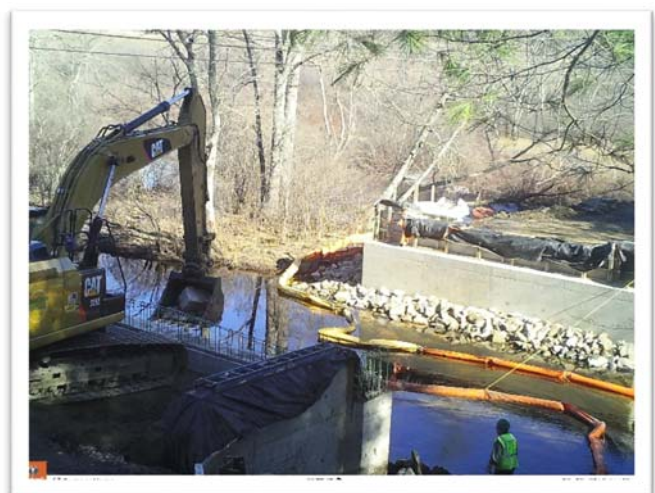
Installing Stone Fill in Front of West Abutment Looking Upstream/North
