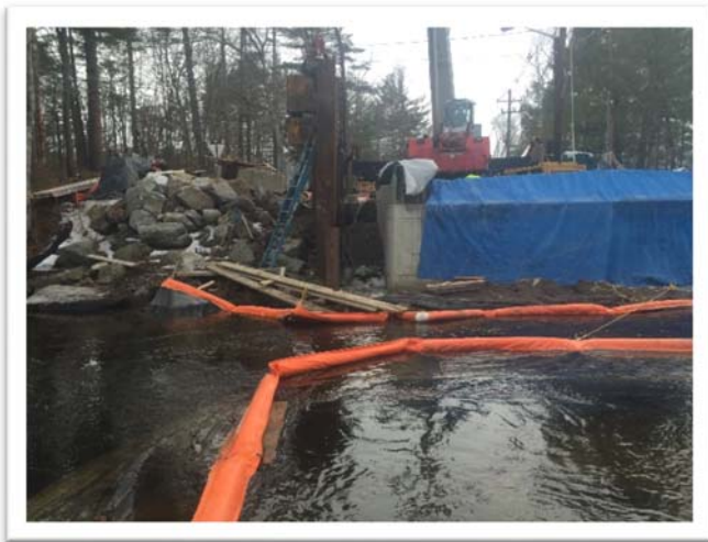
Removing the Cofferdams From the West Abutment Looking West
