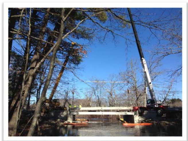
Erecting the 1 st Downstream Exterior Beam Looking Upstream/North
