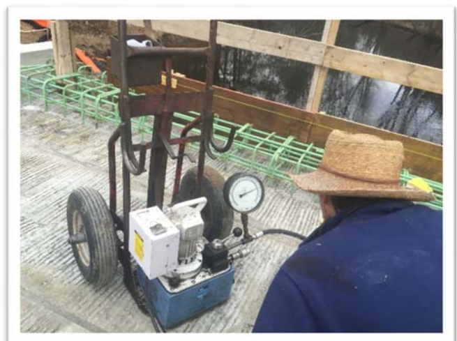
Final Post-Tensioning of the Concrete Beams
