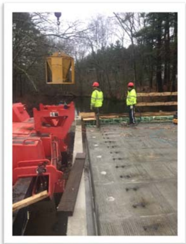
Pouring the Concrete for the Curtain Walls Looking Downstream (South)
