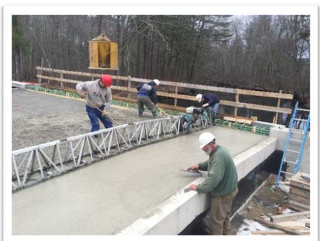
Pouring Concrete Overlay over the Concrete Beams Looking Downstream (South)
