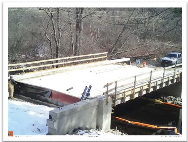
Installing Waterproofing Membrane Behind West Abutment- Looking Upstream (North)
