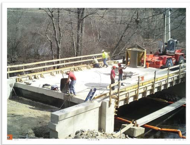
Pouring Concrete Brush Curbs over the Concrete Beams Looking Upstream (North)
