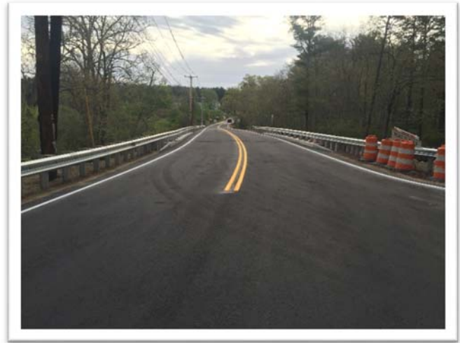
Completed Pavement Markings – Looking East Towards the Bridge
