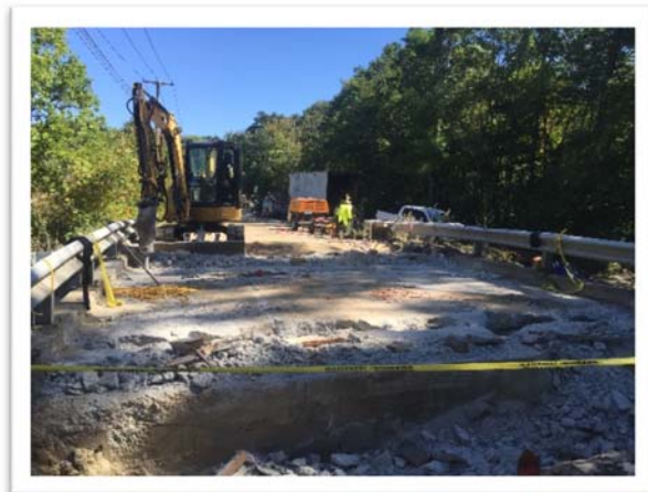
Existing Bridge Deck Removal
