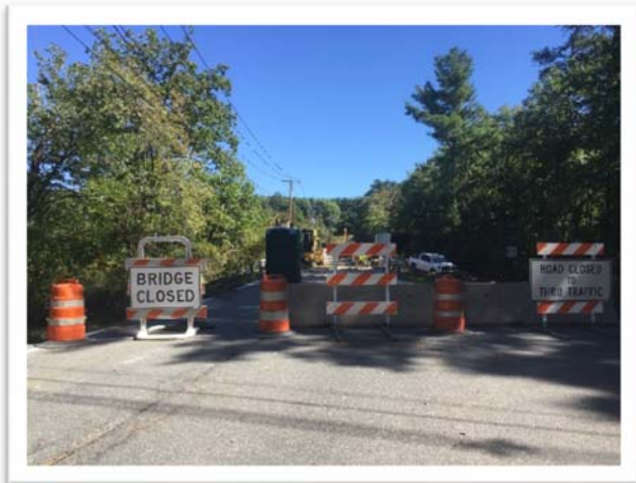
Bridge Closed to Traffic
