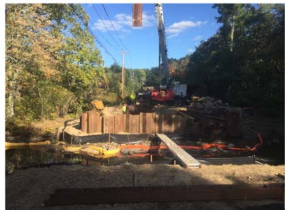
Cofferdam Installation at New East Abutment
